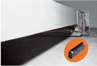
The light barriers are installed on each mobile rack and on the outer sides of the blocks in front of the entryways into the aisles.
